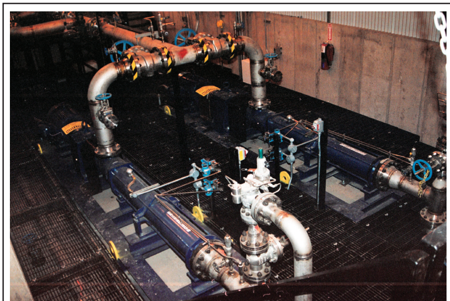
The PCP pumps at the Anschutz Ranch Field handle natural gas condensates and produced water. All wetted metal parts are duplex stainless steel, and the pumps are equipped with a special dry-run protection device.
